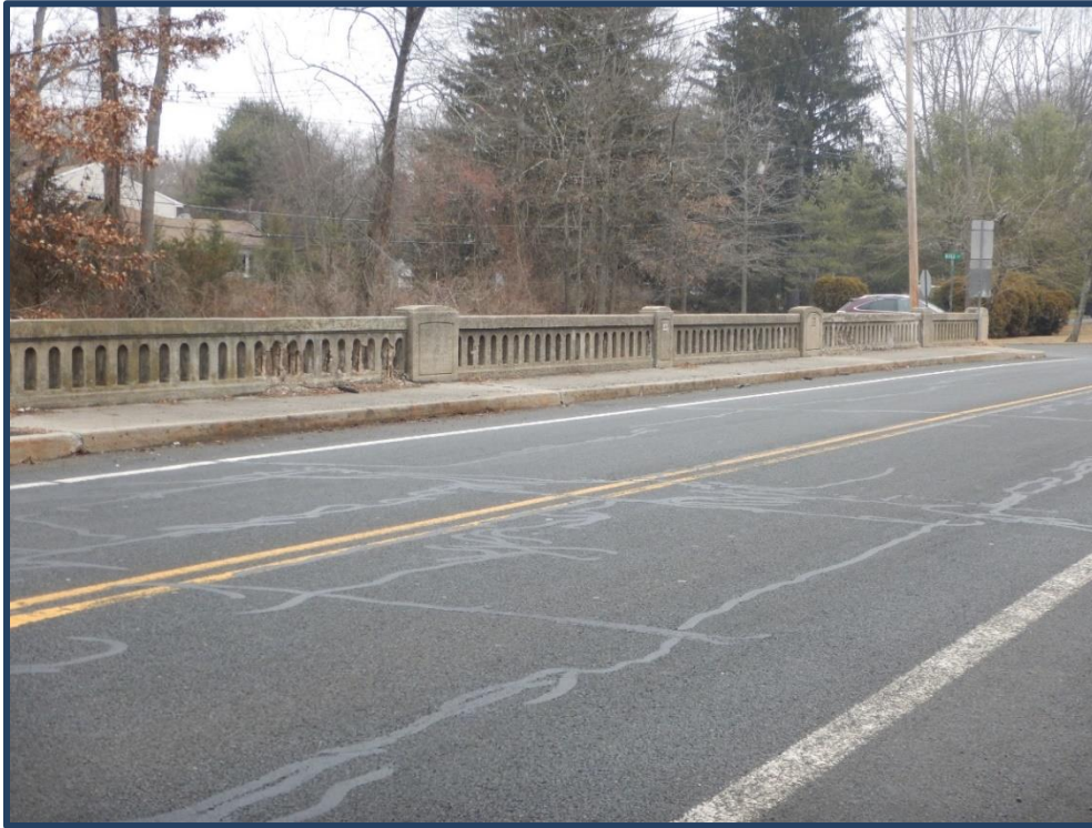
Top of deck, looking northeast
