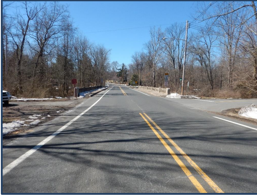
Valley Road east approach to bridge, looking west
