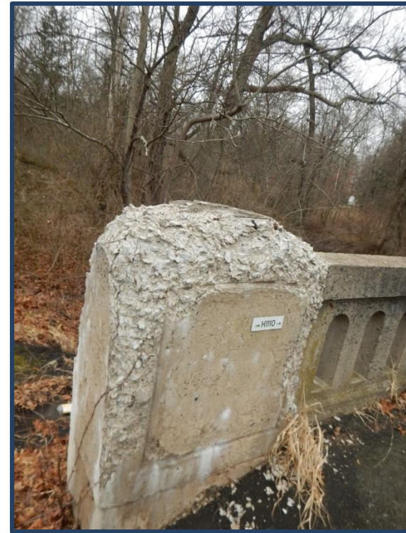
Concrete Pylon @ southeast corner
