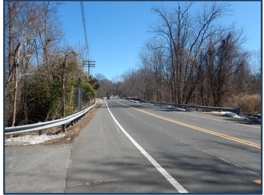
Valley Road west approach to bridge, looking east
