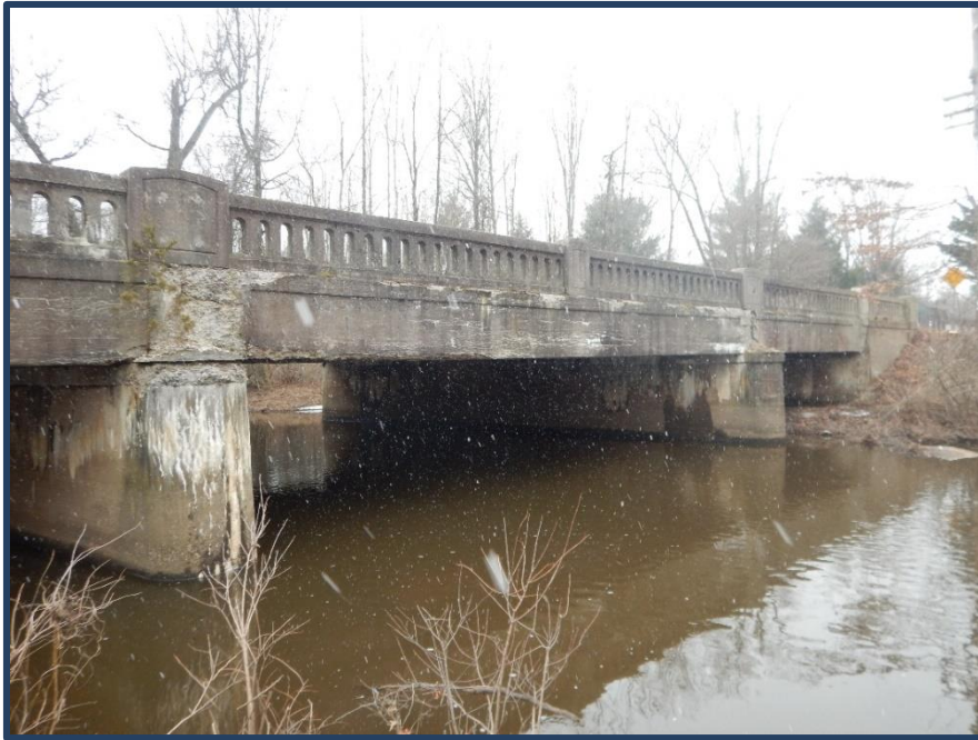
North fascia, looking southwest
