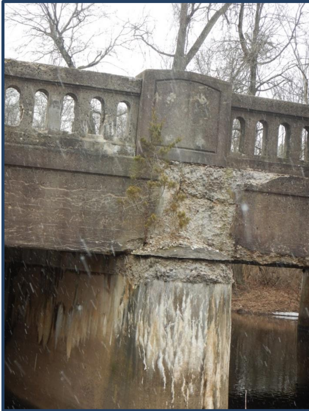
North fascia @ east pier
