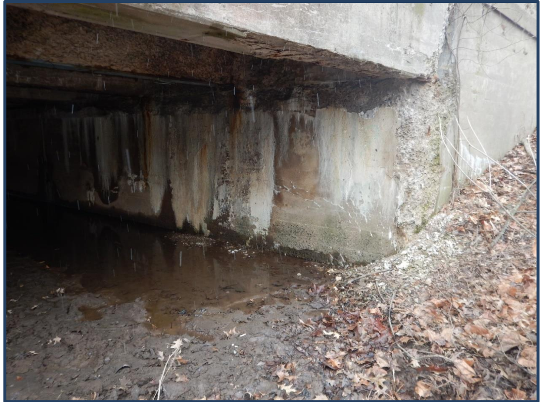
West abutment, looking southwest
