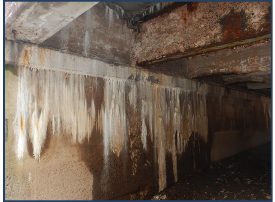
Under bridge, looking at north pier
