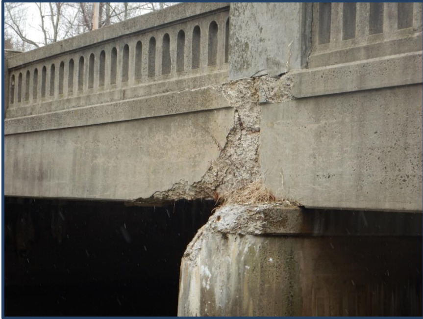
South fascia @ east pier
